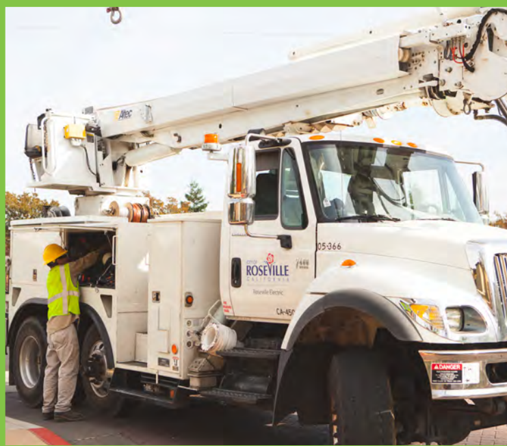
Line truck preparing for utility pole installation
