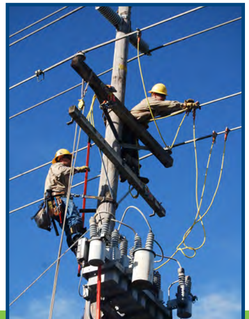
Roseville Electric Utility linemen grounding 12 kV circuits prior to maintenance
