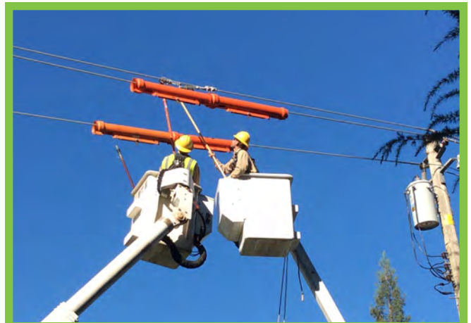
Utility linemen installing protective covers on 12kV system
