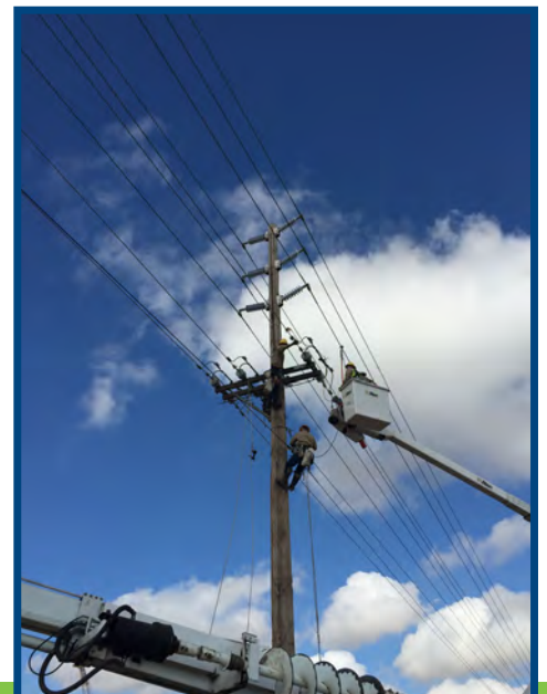
Utility crews performing maintenance on 12kV overhead air switch
