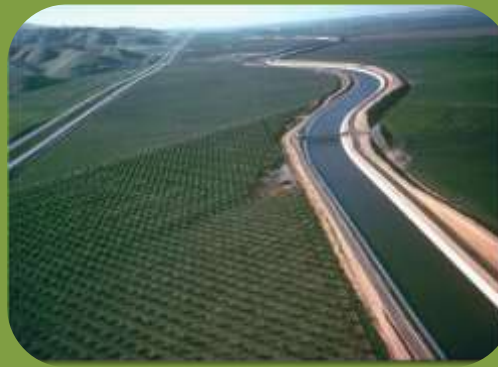
State Water Project
